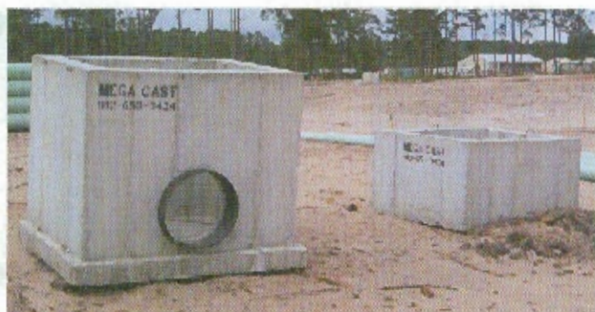
Precast structures awaiting installation
